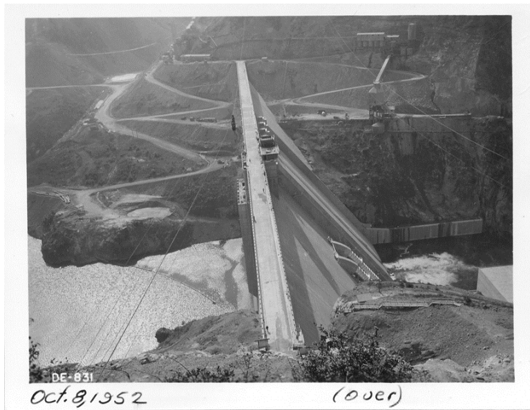
Figure 3-9. View of Left Abutment Construction Fills
