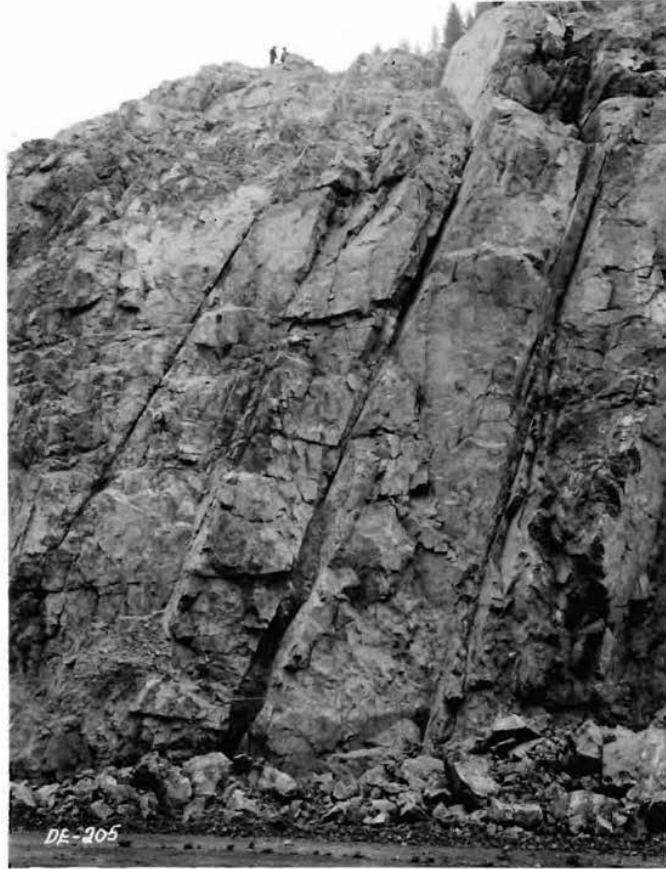
Figure 3-10. Dominant Joint System Set – Right Abutment Highway
