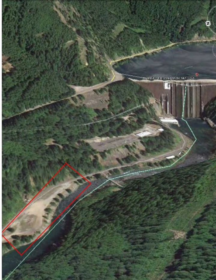
Figure 14-4. Detroit Dam Operations Yard
